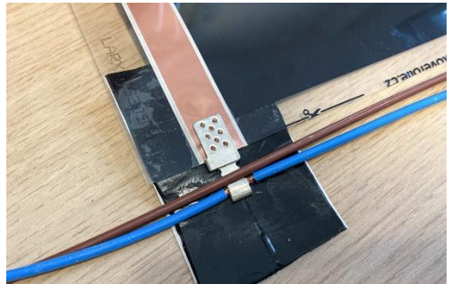
Bottom insulation of connectors
